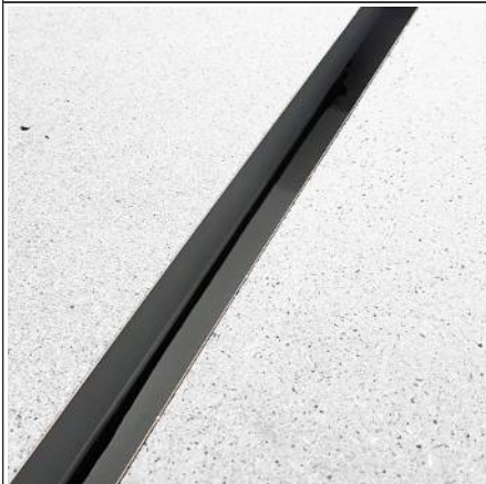
Fig. 10: Plenum box flush in the floor
