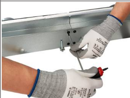
Fig. 7: Screwing the plenum boxes together
