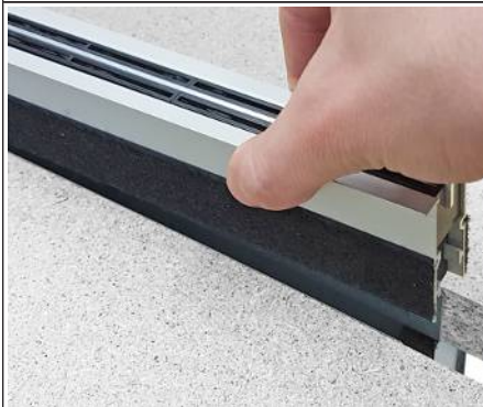
Fig. 11: Inserting the slot outlet
