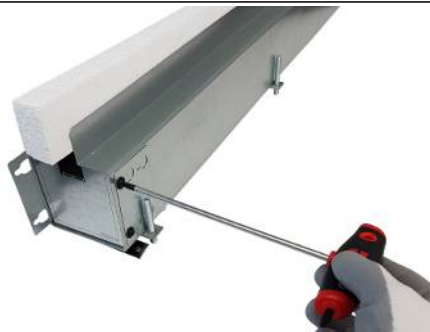
Fig. 6: Loosening the screws of the connecting panel
