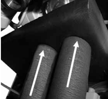
Fig. 41: Fix insulation through the openings of the condensate tray
